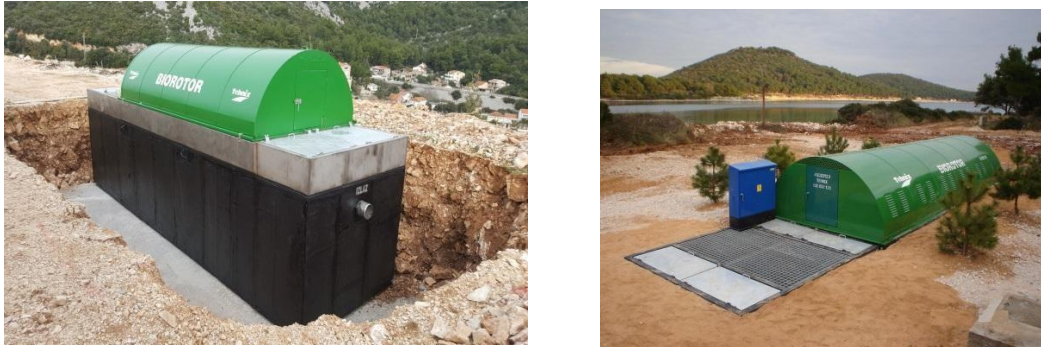
Fig. 6. Practical construction of Biorotor Tehnix 200
